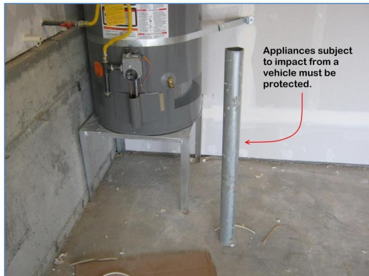
Figure 3 Water heater protect
